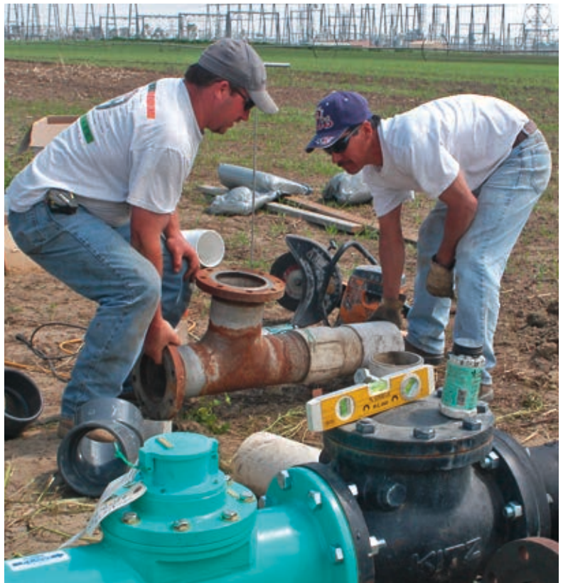
Meter and line replacement on an agricultural well in Chino Basin.
