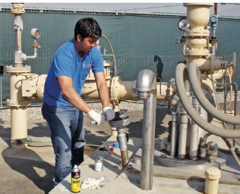
At work on a desalter well.
